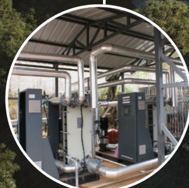
Air Compressor Heat Recovery System
